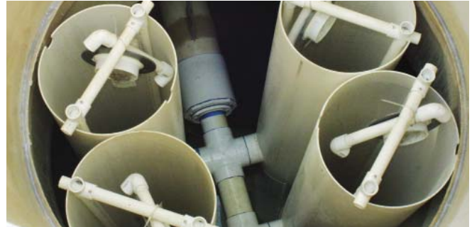
Filter housings were fabricated and assembled before shipping to the tank installation site.
